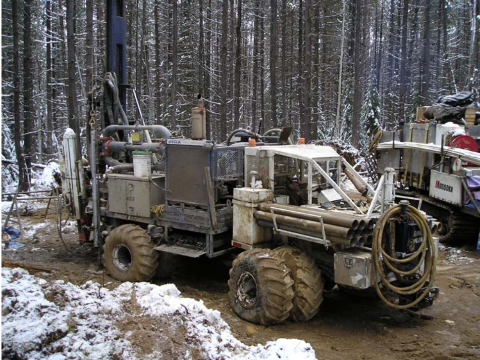
Photo I-3 Skidder mounted drill rig
