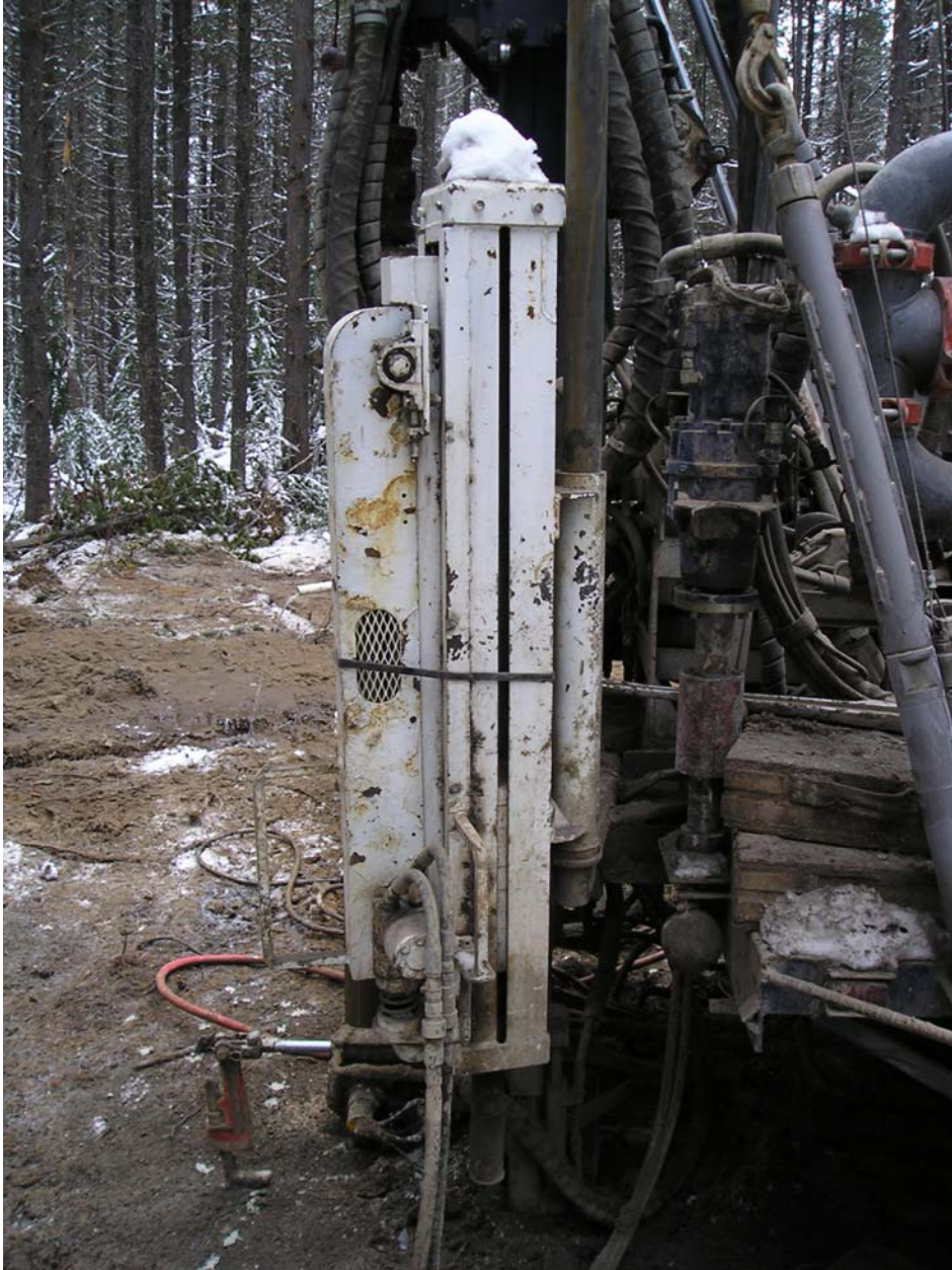
Photo I-5 Automatic trip SPT hammer
